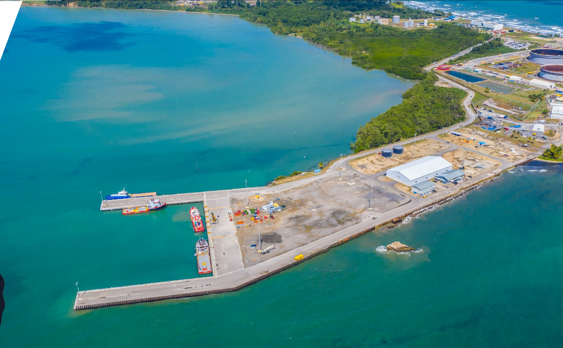
Aerial View of National Energy's Port of Galeota Facility, Guayaguayare
