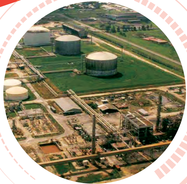
Aerial view of methanol and ammonia plants at Point Lisas Industrial Estate, 2001.
