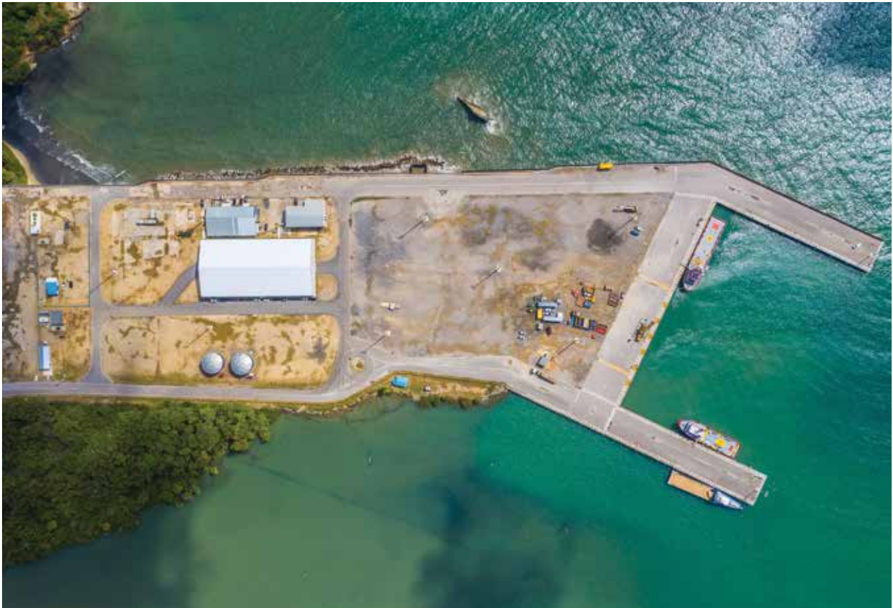
Aerial view of the Port of Galeota
