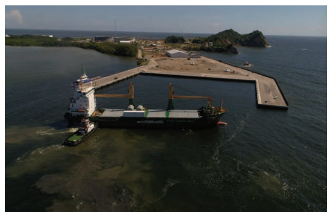
National Energy tug assists vessel berthing at the Port of Galeota
