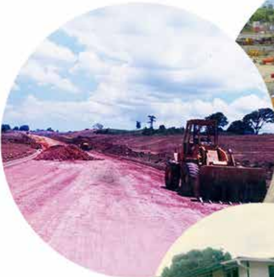
Construction of La Brea Industrial Estate, 1996
