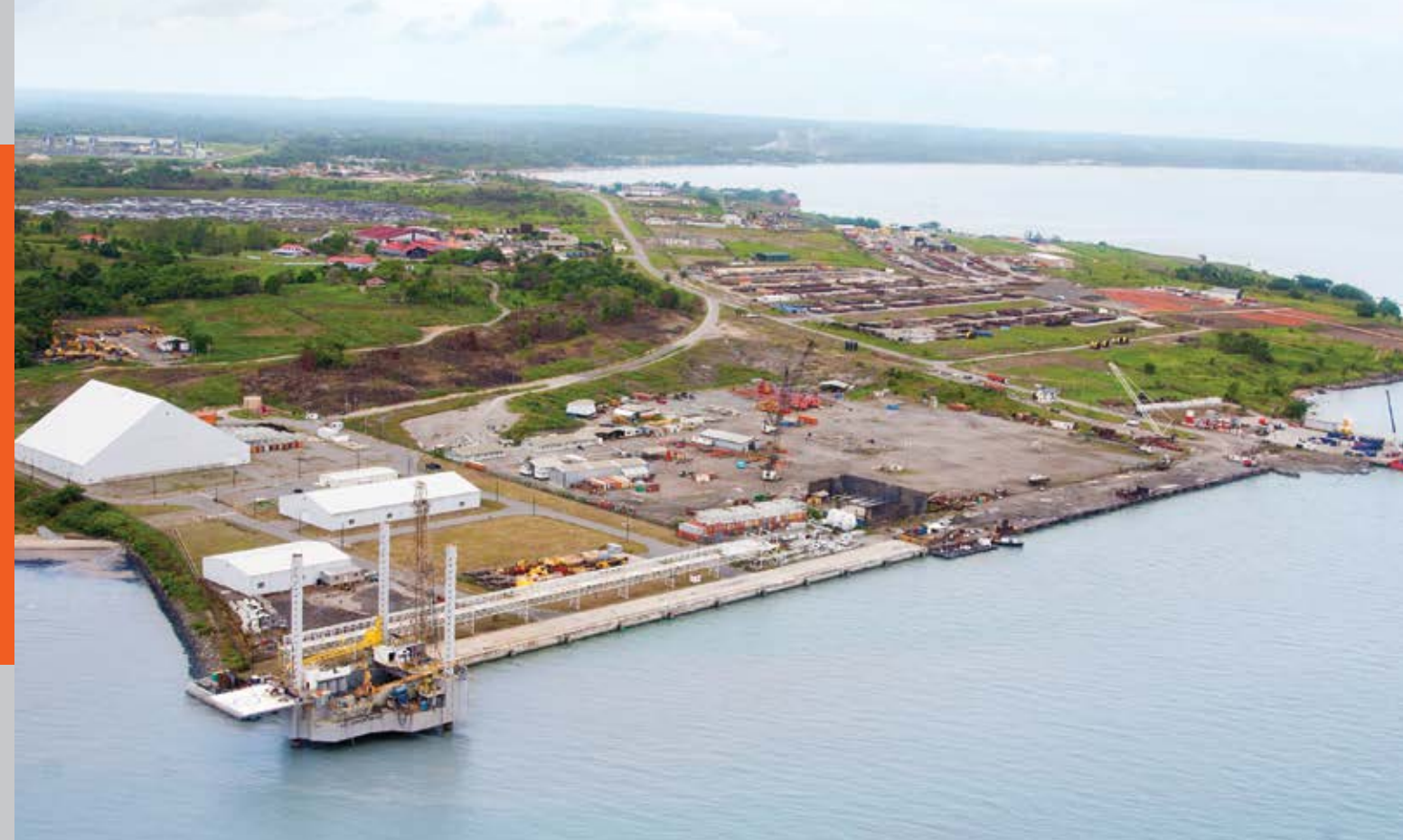
Figure 3: Aerial View of Berths and Fabrication Yard at LABIDCO (2013).
