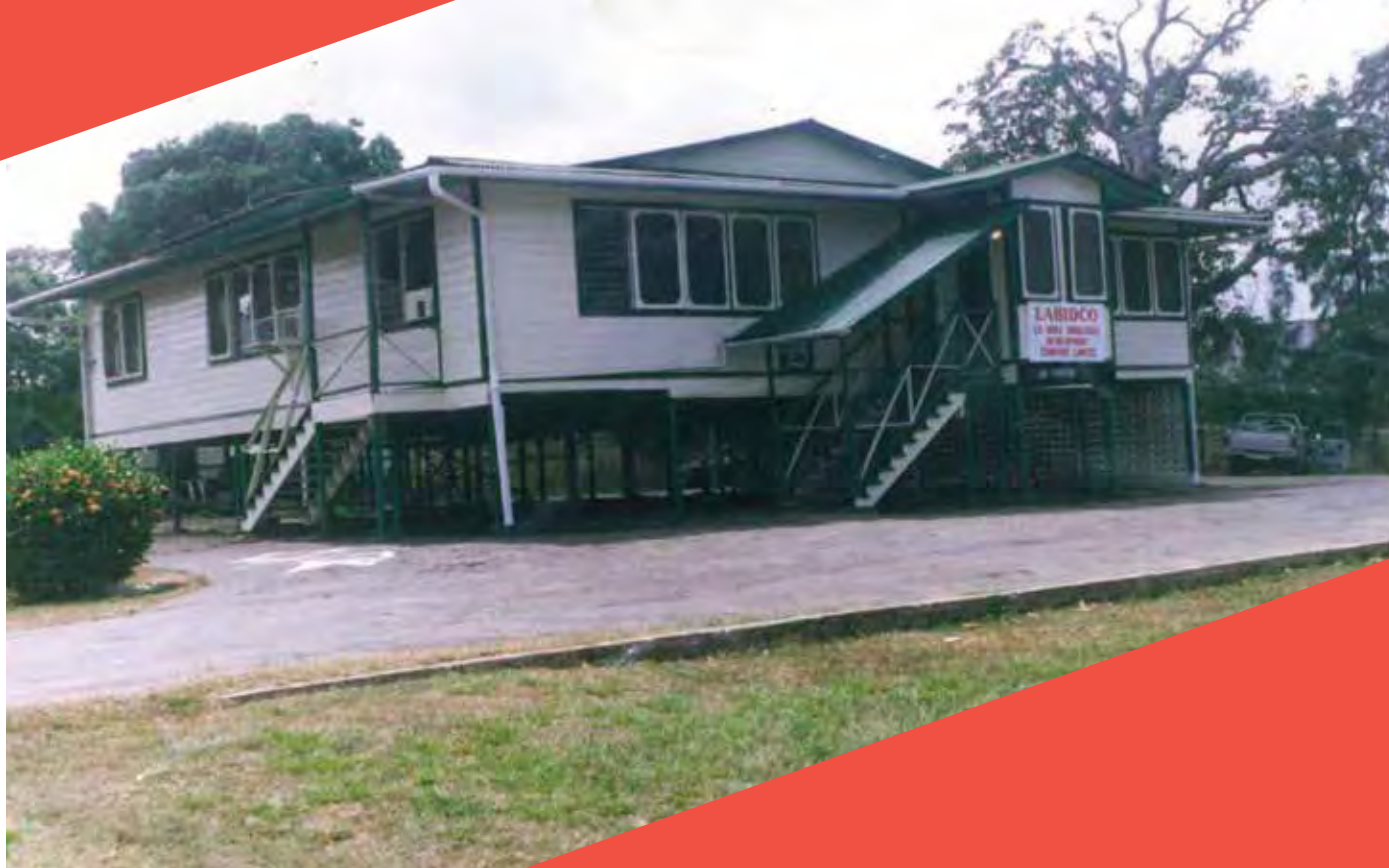
LABIDCO's first office building, Bungalow 14
