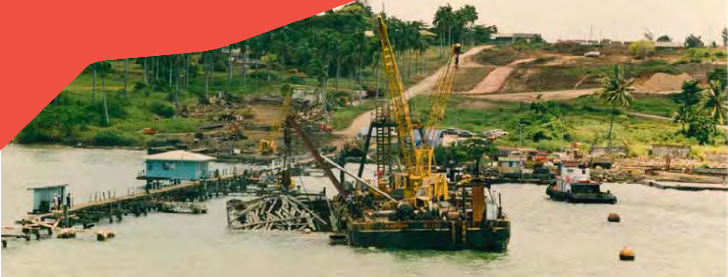
Demolition of Brighton Jetty, 1993
